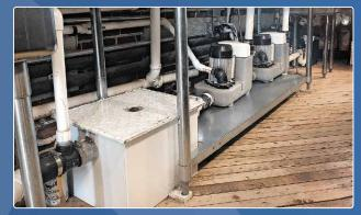
A 1-inch PVC drain line is connected to a three-bay sink and dishwasher situated to the right of the pump trio. This drain line first runs into a grease trap before connecting to one of the Sanicom 1 units.
