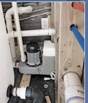
The Sanicom 1 drain pump showing the 1-inch discharge pipe running vertically to discharge the gray water from the washing machine into the blackwater tank. The washing machine will drain into the Sanicom 1 via a 2-inch inlet (on the left).
