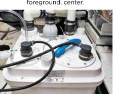
Inside the RV MANTA's mechanical room, showing the Sanicubic 1 and the 1.5-inch PVC piping to two of the Sanicubic 1's four input ports.
