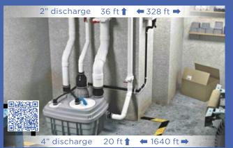
Discharge rate at 36' (2"): 26 gal/min (136 liters/min)
