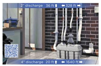
**Discharge rate:** (Both motors in operation) at 36' (2"): 40 gal/min (151 liters/min) at 3' (2"): 145 gal/min (549 liters/min) at 20' (4"): 110 gal/min (416 liters/min) at 3' (4"): 250 gal/min (946 liters/min)
